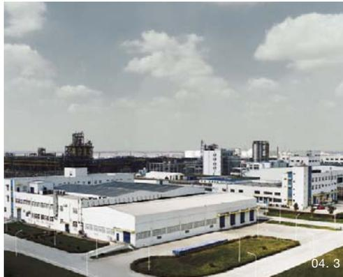
benefit for WACKER is that the sheer size of the plant reduces production and infrastructure costs. Dow Corning in turn benefits from WACKER's vast experience with the pyrogenic silica production process. Pyrogenic silica is produced from the waste from siloxane production. This results in a cycle which utilizes 90% of all by-products, which would otherwise require disposal.
